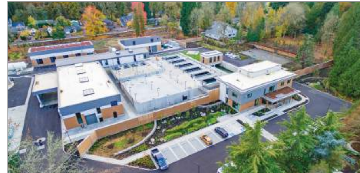
Photo: Lake Oswego Tigard Water Treatment Plant.
