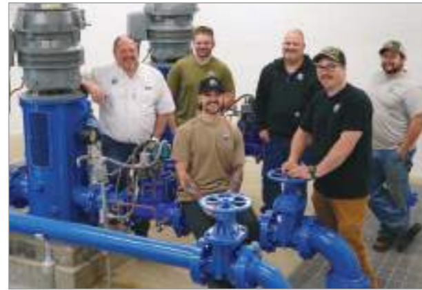
The City's Water distribution team at the new 10th Street pump station.
